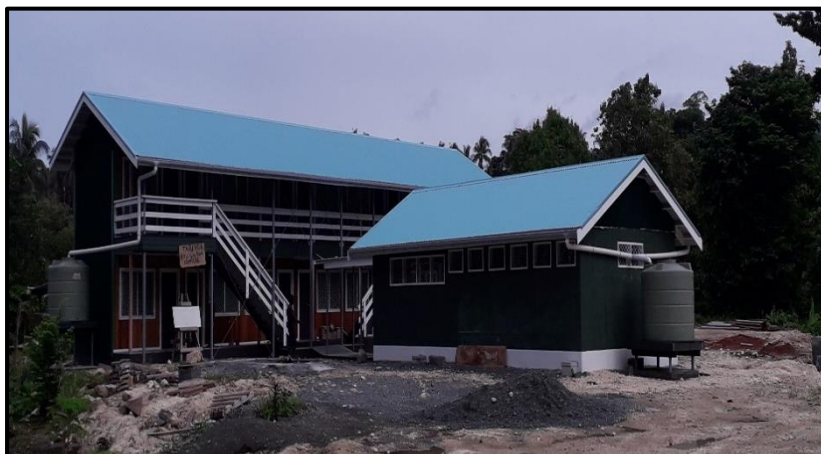
Completed Girls Dormitory and Ablution Block at Papara CHS, Choiseul.
