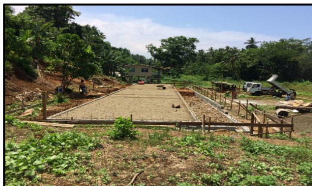
Classroom Building Project at Ngonihau PS, Makira at the foundation stage
