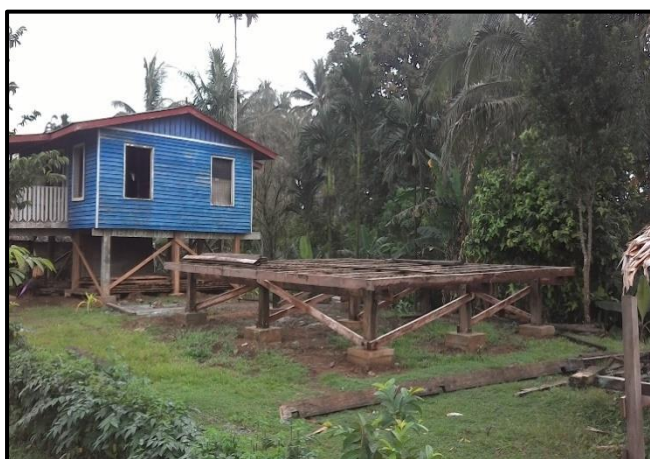
Staff Houses repaired at Warohinou PS, Makira.
