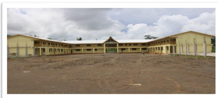
Figure 8: Garanga new classroom building in Isabel Province
